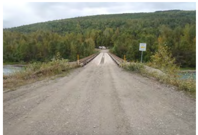
Figure 1-4: Looking towards Wells end.
