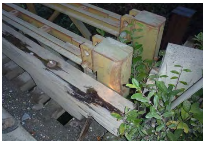
Figure 1-15: Typical impact damage to end post, Wells end upstream shown.
