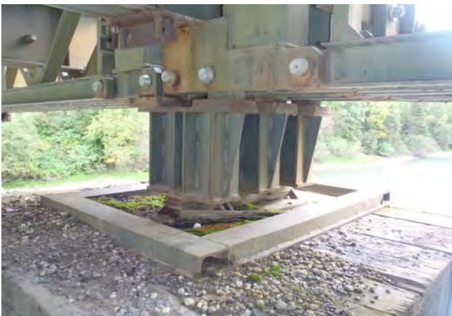
Figure 1-29: Typical pier bearing condition, Pier 2 downstream shown, note debris accumulation.
