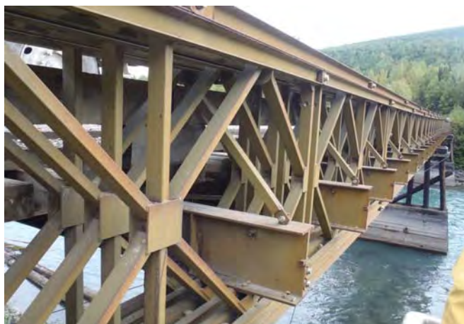
Figure 1-12: Typical panel condition, span 3 downstream shown.
