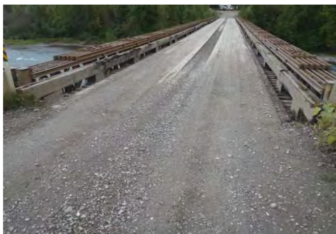
Figure 1-7: Likely end abutment deck end.
