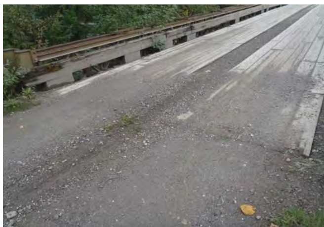
Figure 1-8: Wells end abutment deck end.
